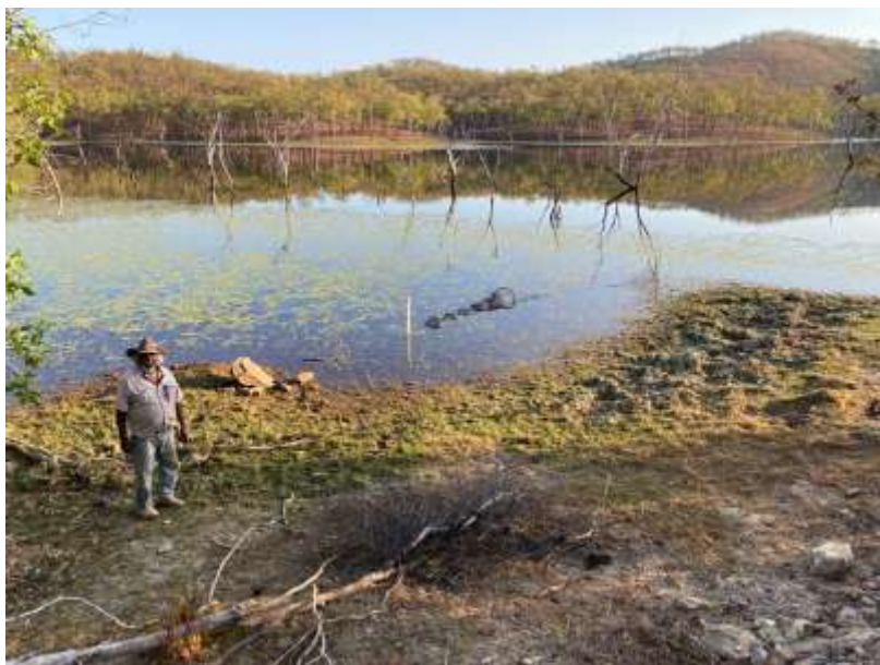
Figure 1 - Danny at Raw Water Dam 1 (note fauna trap in the water)
